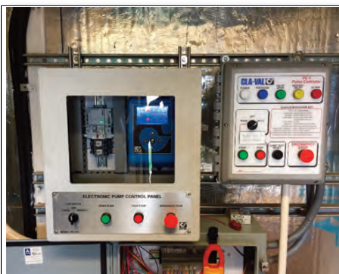
Electronic Pump Control with the PC-22D
